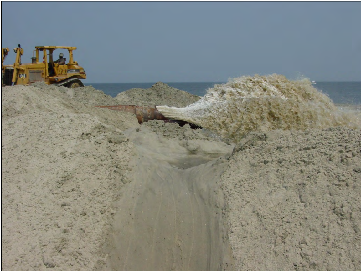
Figure 5-1. Example of Beach Fill Being Constructed
